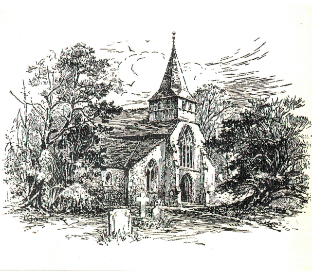
Buckland Church, Dover
